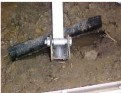
Poor site grading led to loose strap
