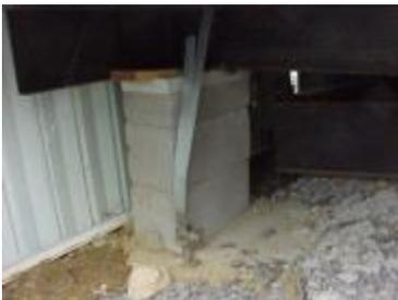
This is NOT proper anchoring!
