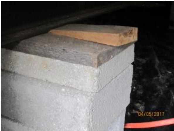
Check your installation manual to make sure you are using the proper cap and spacer material.
